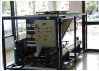
Chillers and cooling units
